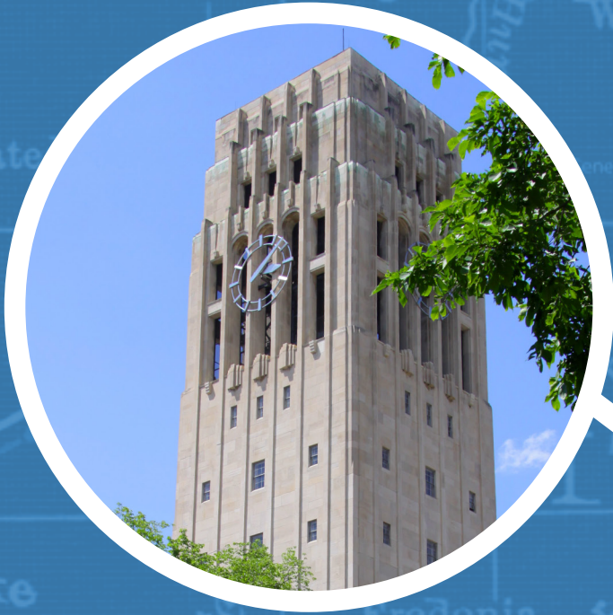
Burton Memorial Tower Ann Arbor, MI
